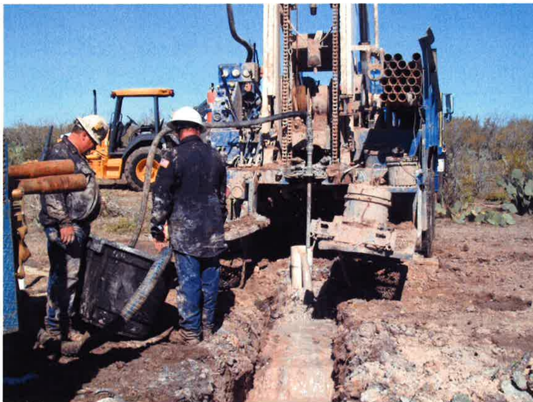
Photo 3 - Grouting Boring B-52 – January 2015
